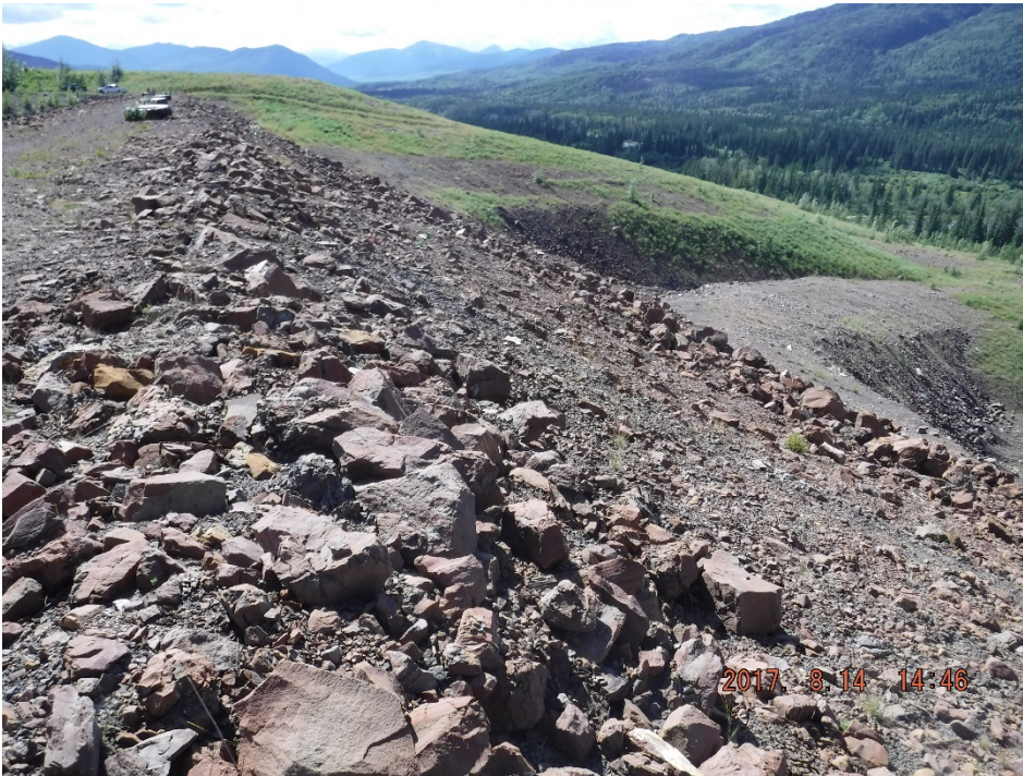
Photo I-5 Downstream slope – looking southwest. No sign of erosion or significant movement (SNTD-2017-03)
