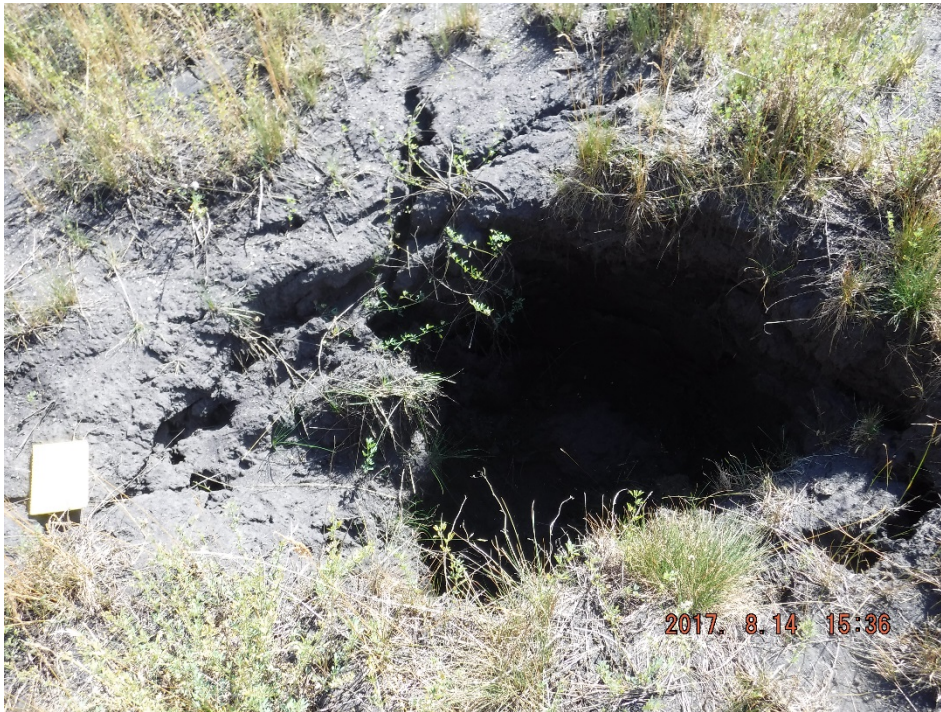
Photo I-15 Sinkhole 1 – first observed in 2016. Approximately 1.2 m x 1.9 m x 1.0 m deep (SNTD-2017-11)
