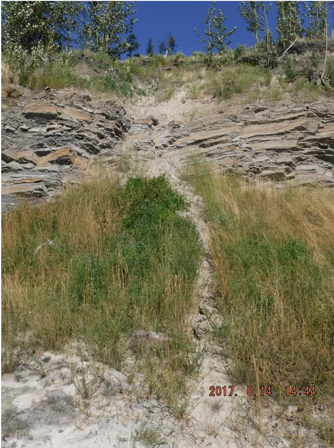
Photo I-4 East abutment – minor ravelling of material from slope above onto the crest – appears to be in the same condition as previous year (SNTD-2017-02)
