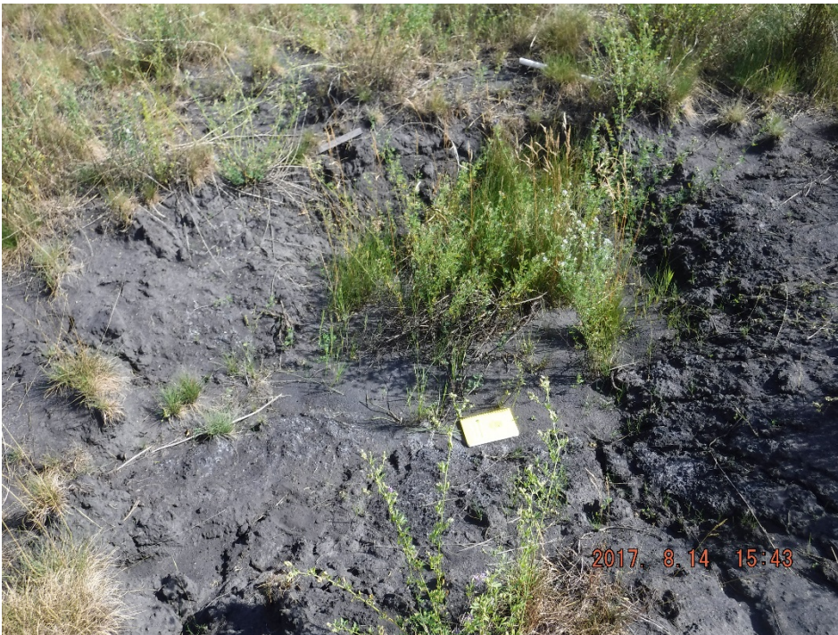
Photo I-17 Sinkhole 3 – approximately 2.5 m x 2.3 m x 0.5 m deep (SNTD-2017-13)
