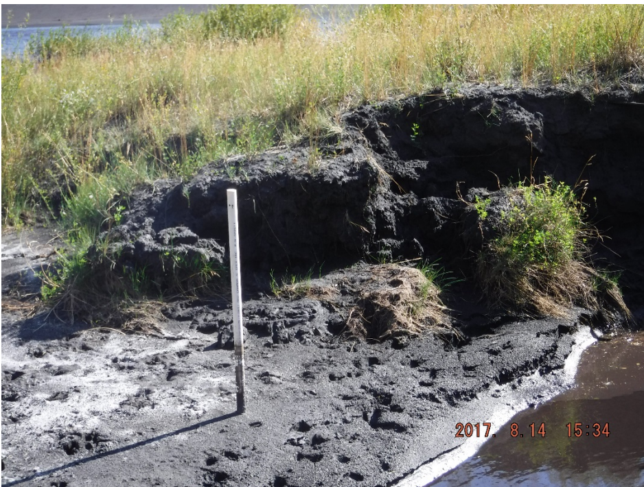
Photo I-14 Offshoot of main drainage channel – closeup view of the slumping (SNTD-2017-10)
