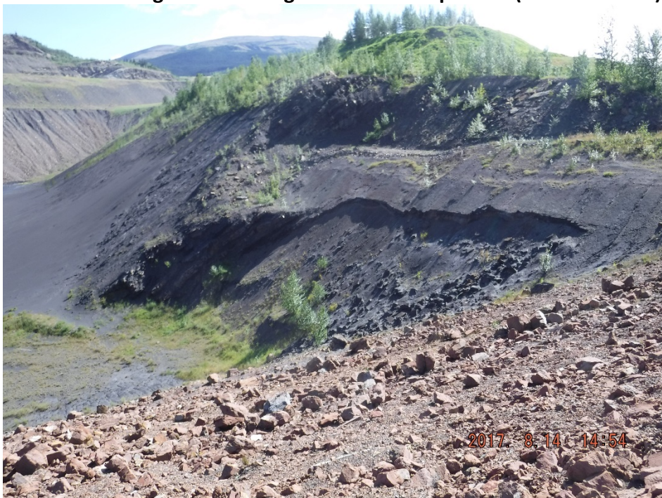
Photo I-8 West abutment, continued ravelling of shale slope upstream of abutment. No significant change from 2016 inspection (SNTD-2017-06)
