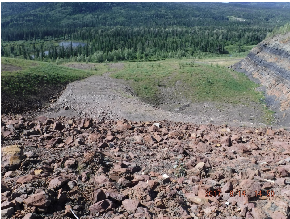
Photo I-6 Downstream slope taken from mid-length of the crest – slope appears to be in good condition (SNTD-2017-04)
