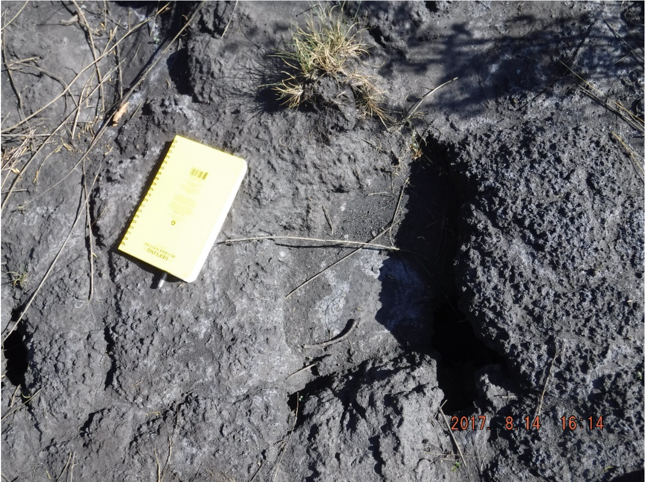
Photo I-26 Sinkhole 9 – first observed in 2016. Approximately 0.1 m x 0.1 m x 0.1 m deep (SNTD-2017-20)
