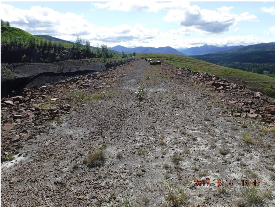
Photo I-3 Dam crest from east abutment – no sign of movement or settling (e.g., sinkholes, cracks, slumping) (SNTD-2017-02)
