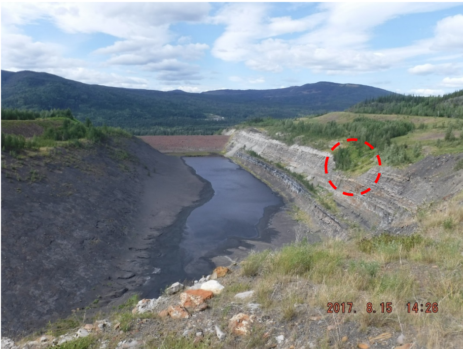
Photo I-31 Shikano North Tailings Dam – looking south. Historic slumping failure circled with red dash line. No significant change since 2012 (SNTD-2017-24)
