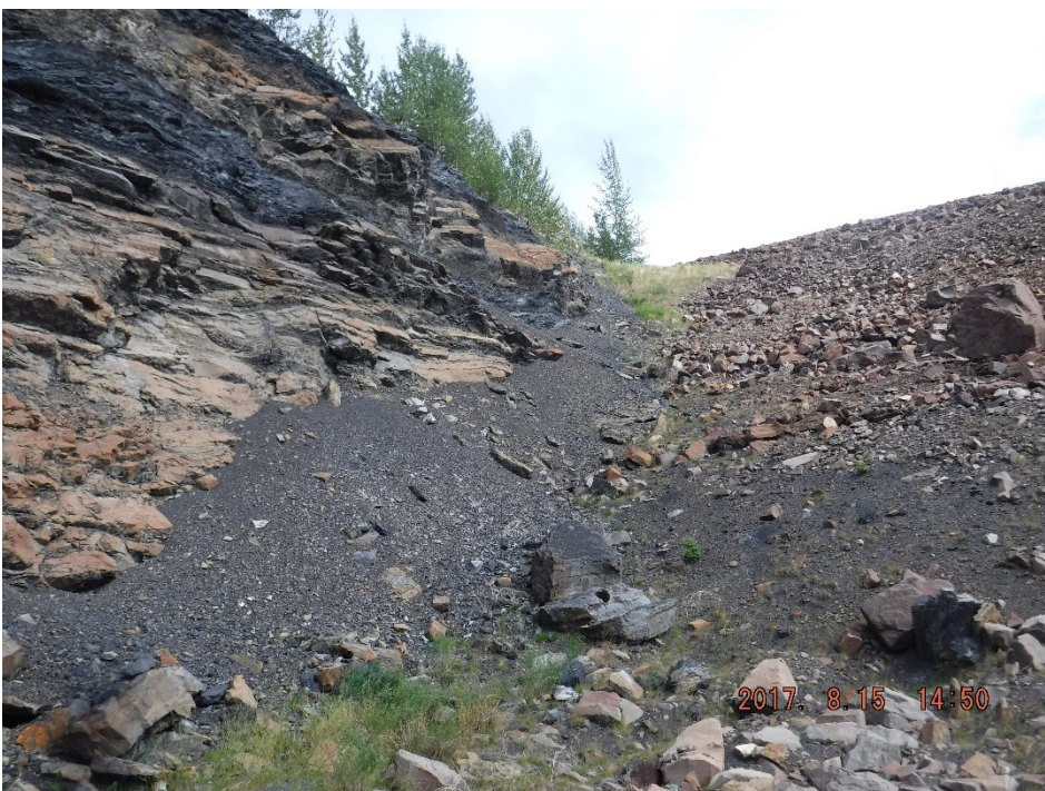
Photo I-33 Downstream contact with east abutment – no change in condition from previous year (SNTD-2017-26)
