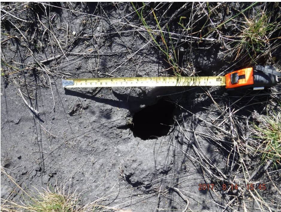
Photo I-18 Sinkhole 4 – was not observed in 2016. Approximately 0.2 m x 0.1 m x 0.7 m deep (SNTD-2017-14)
