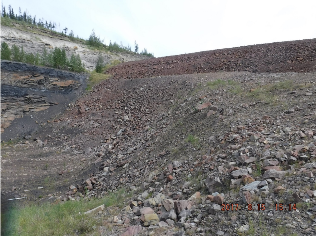
Photo I-34 Downstream, access ramp and downstream slope – no significant sign of erosion or movement (SNTD-2017-27)
