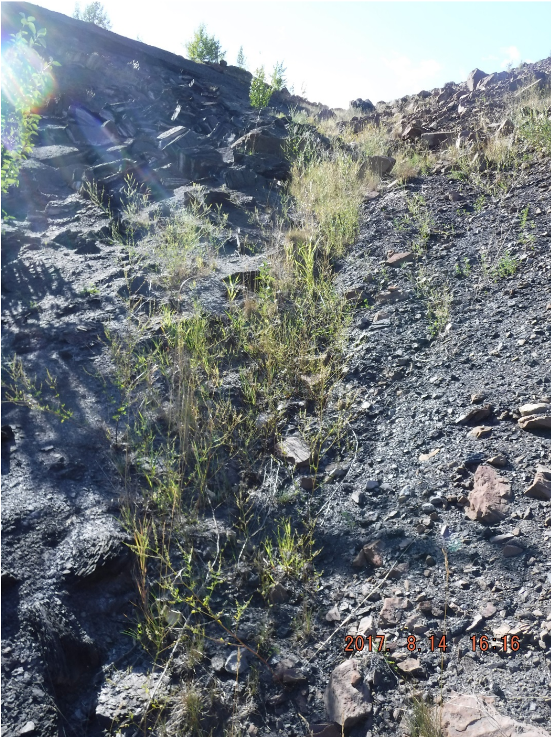
Photo I-27 SNTD west abutment - upstream contact with the Shikano pit west wall – small erosion gully noted (SNTD-2017-21)
