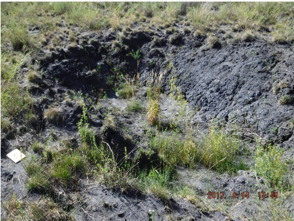
Photo I-22 Sinkhole 6 - partial view of sinkhole cluster. Approximately 3.5 m x 6.7 m x 0.9 m deep (SNTD-2017-16)
