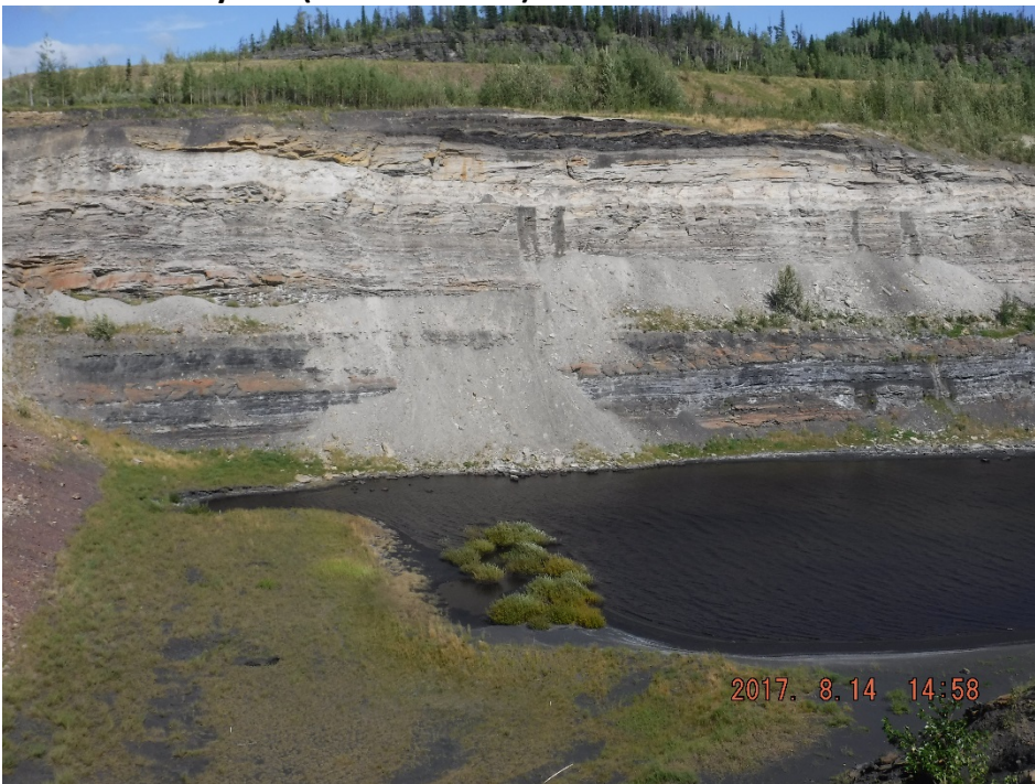
Photo I-10 North abutment – looking northeast; erosion appears unchanged from previous years (SNTD-2017-07)
