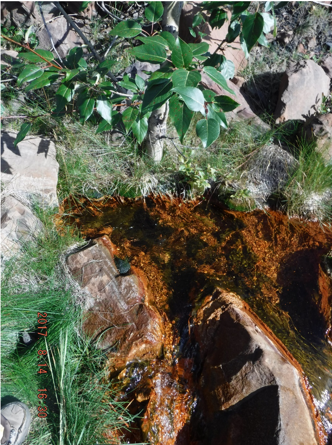
Photo I-28 Seepage from low level outlet downstream of the dam (SNTD-2017-22)
