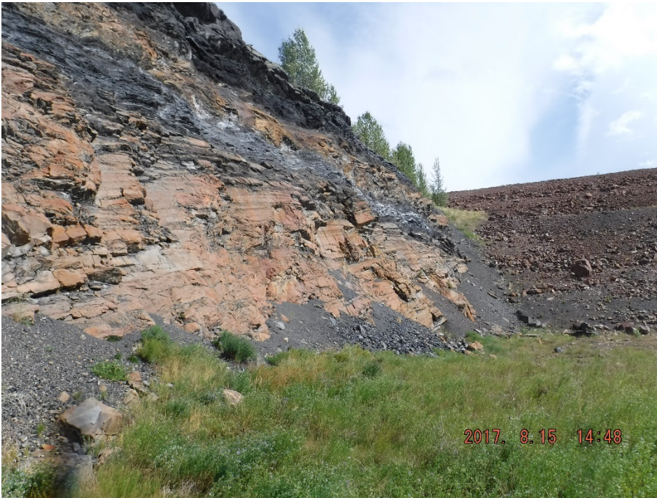
Photo I-32 Downstream east abutment – looking southeast. No change in condition from previous year (SNTD-2017-25)
