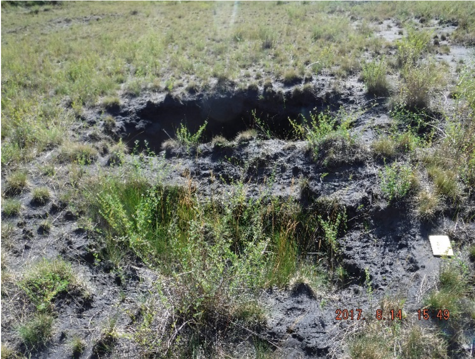
Photo I-21 Sinkhole 6 - partial view of sinkhole cluster. Approximately 1.2 m x 1.3 m x 0.5 m deep (SNTD-2017-16)
