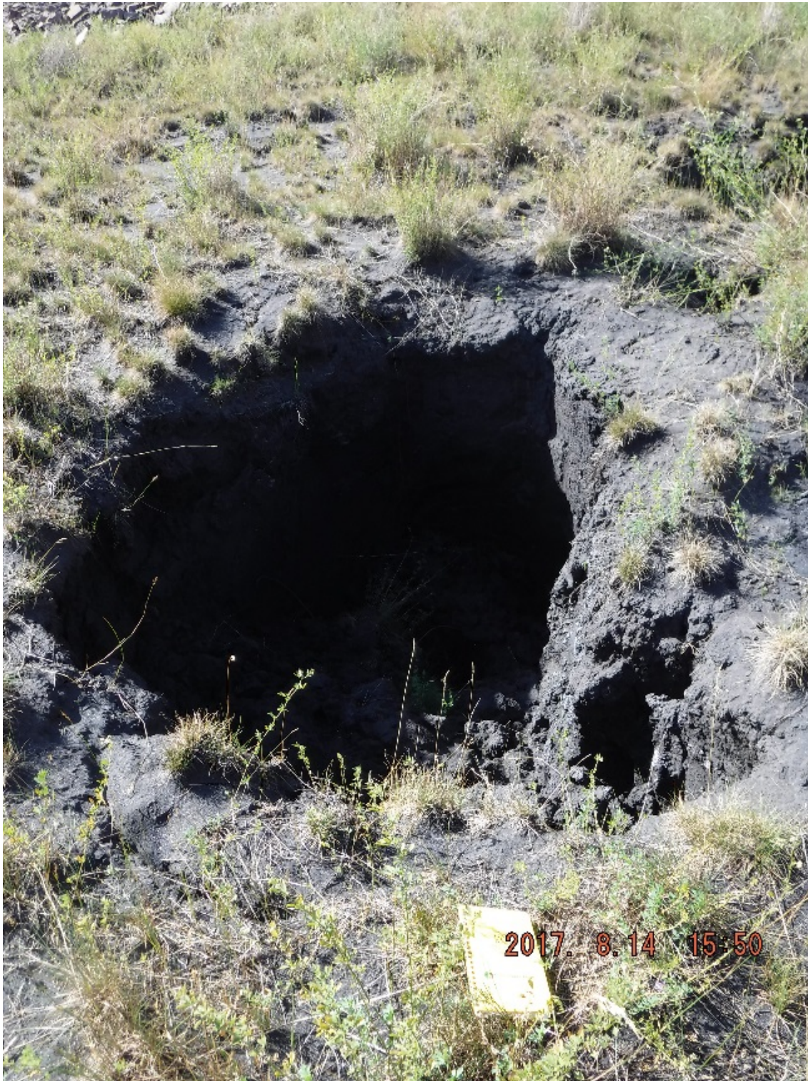
Photo I-23 Sinkhole 6 - partial view of sinkhole cluster. Approximately 1.9 m x 3.2 m x 1.9 m deep (SNTD-2017-16)
