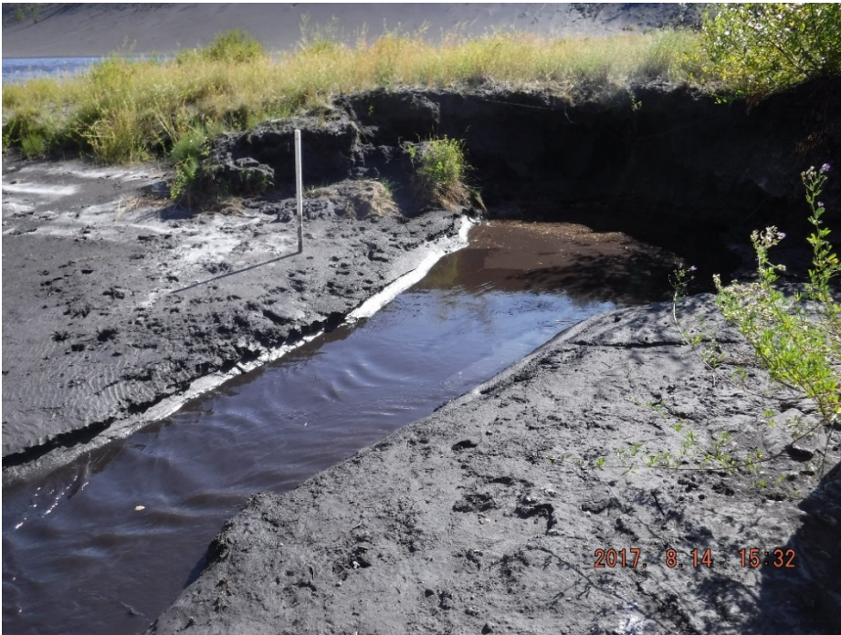
Photo I-13 Offshoot of main drainage channel from the tailings pond to the upstream face of the SNTD; signs of slumping within tailings around the channel. (SNTD-2017-09)
