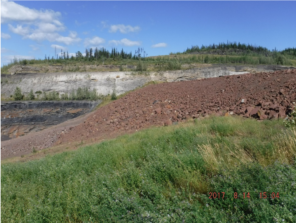
Photo I-11 Downstream slope taken from west abutment – looking northeast; no sign of erosion or movement (SNTD-2015-08)
