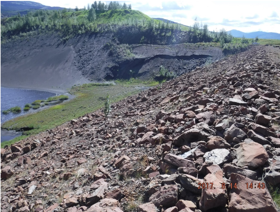
Photo I-2 Upstream slope – looking southwest. No sign of erosion or movement (SNTD-2017-01)
