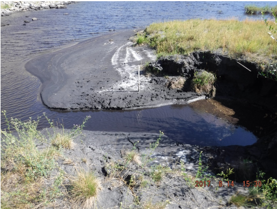
Photo I-12 Drainage channel inside the impoundment (SNTD-2017-09)
