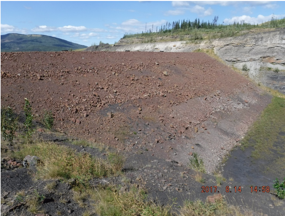
Photo I-9 Upstream slope taken from the west abutment – looking northeast. Slope appears to be in good condition with no significant sign of erosion or movement (SNTD-2017-07)
