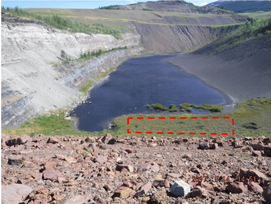
Photo I-8 West abutment, continued ravelling of shale slope upstream of abutment. No significant change from 2016 inspection (SNTD-2017-06)
