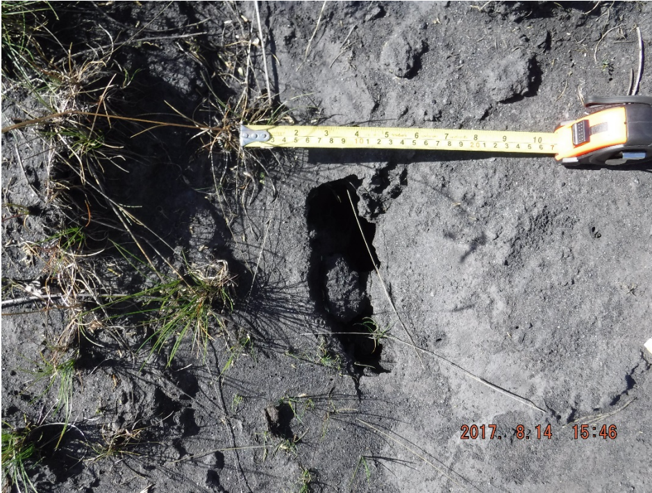
Photo I-19 Sinkhole 5 – was not observed in 2016. Approximately 0.2 m x 0.1 m x 0.2 m deep (SNTD-2017-15)
